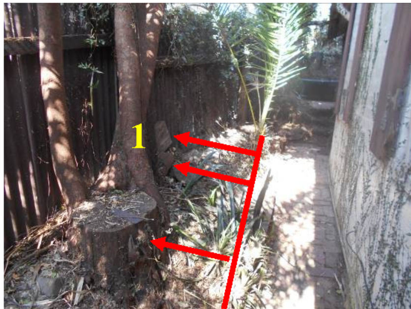
Figure 4 – showing the location of Tree 1 in relation to the existing dwelling. This species is bordered by two properties. This species is located in a raised garden bed before stepping down to a paved area an estimated 30cm below the stump. The area in red is identified as the raised garden bed area. This area will need to be maintained as a protection zone in order to retain the tree.
