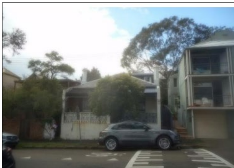
Figure 2: Front elevation from Birchgrove Road. Subject site to left. 101 Birchgrove to right behind street tree with existing first floor. 99 Birchgrove on far right – three storey dwelling.
